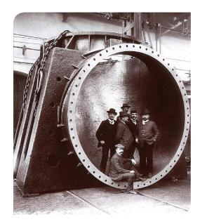
**Right:** A 50t cast-steel piping branch for the hydroelectric power plant at Niagara Falls before it left the Škoda factory in 1905.
